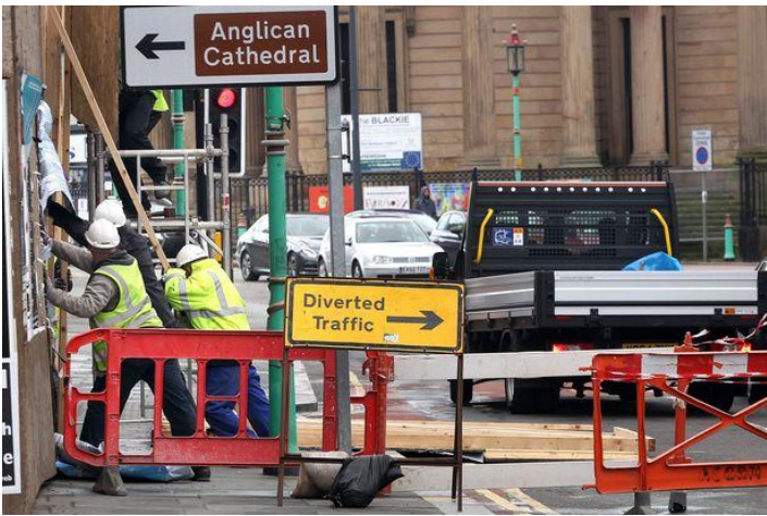
City Centre road closures due to building damage caused by high winds March 2015
