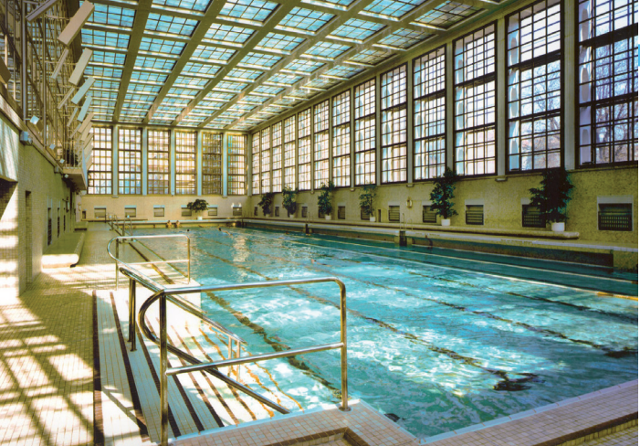
Role model: Public baths in Berlin's Mitte district, which have been refurbished with energy efficiency in mind.
