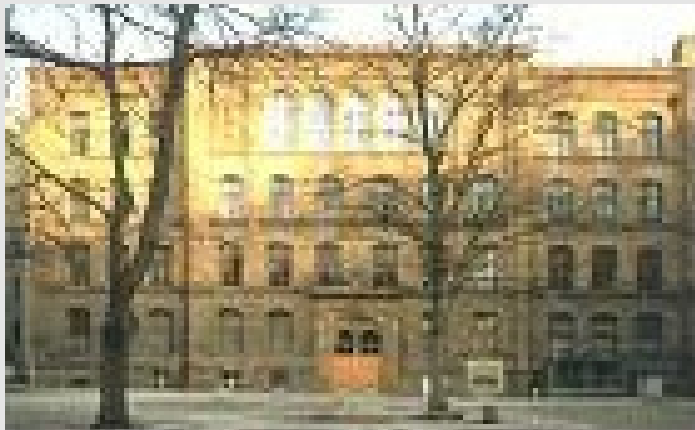
Berlin-Prenzlauer Berg Rehabilitation of a primary school Listed period building
