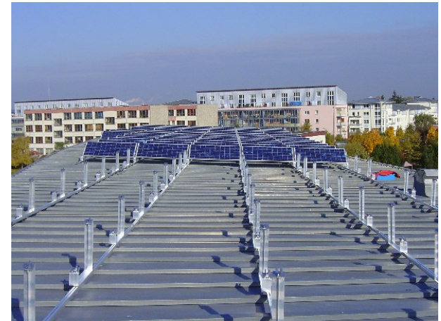
Installation of pv systems on school roof top
